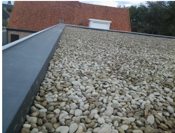
Foto dakplatform in EPDM ter illustratie
