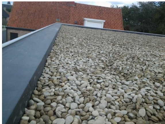
Foto dakplatform in EPDM ter illustratie
