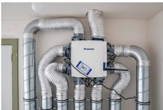
Ventilatiesysteem C+ Healthbox 3.0 Renson
